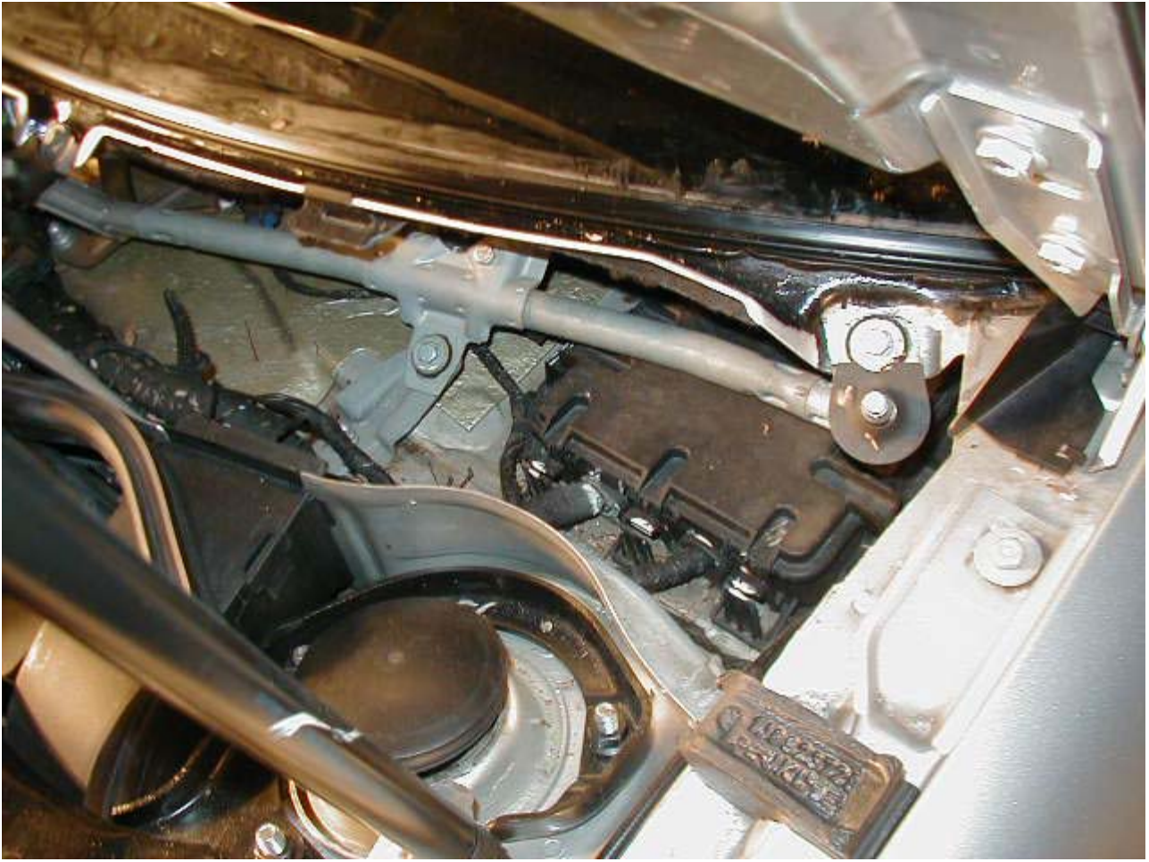
Access to Water-Tight Box
