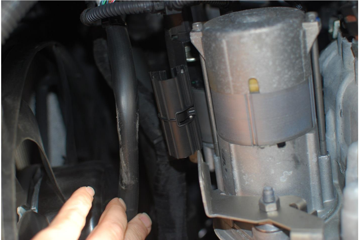
The cable lays in this clip closer to the drivers side of the car. Lifts right out
