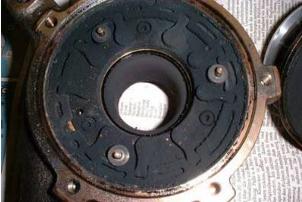
This is a carbon fouled actuator ring mechanism. Fortunately, it can be cleaned rather easily with solvent. Note the three Torx screws that need to be loosened.
